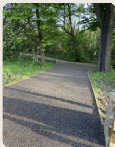
New footway through woodland linking Local Authority routes
