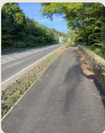
New pedestrian footway that is adjacent to the A616
