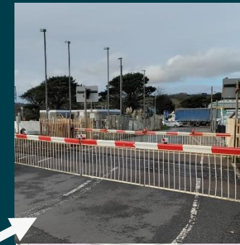
Poniou Lane Level Crossing
