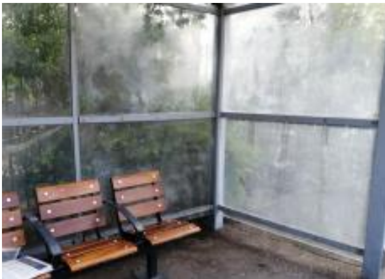
There is a shelter and somewhere to wait for your train, but it is not well maintained
