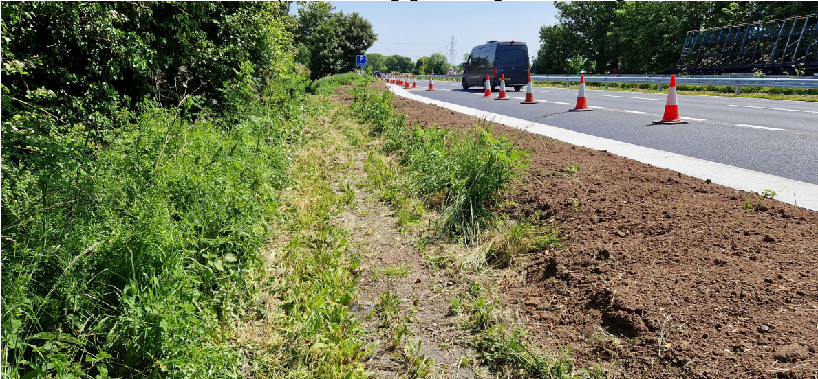
Tarmac path completely buried under vegetation.
