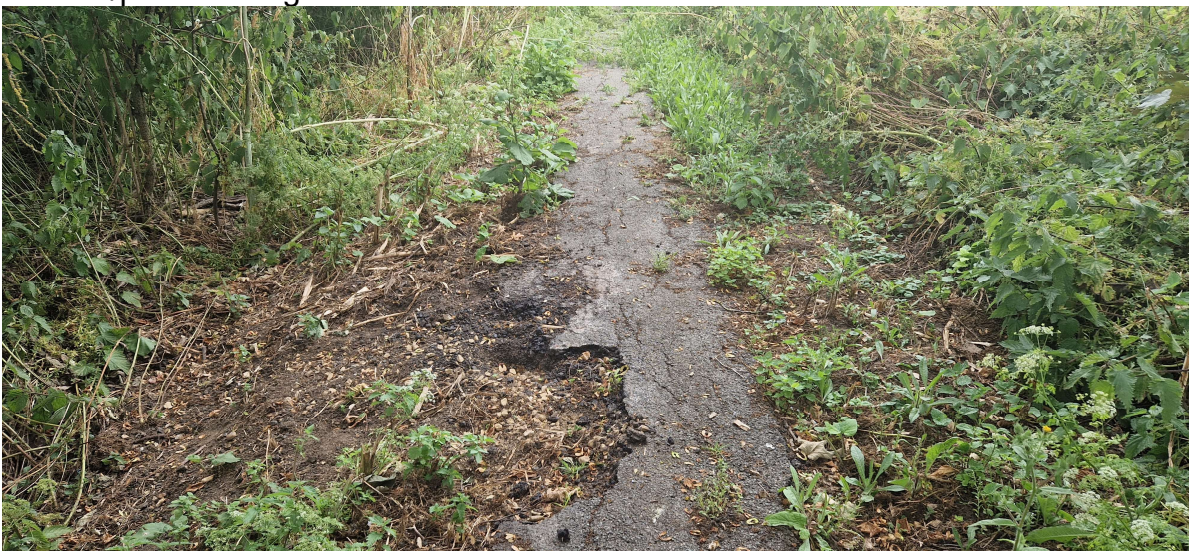
Pothole/path disintegration
