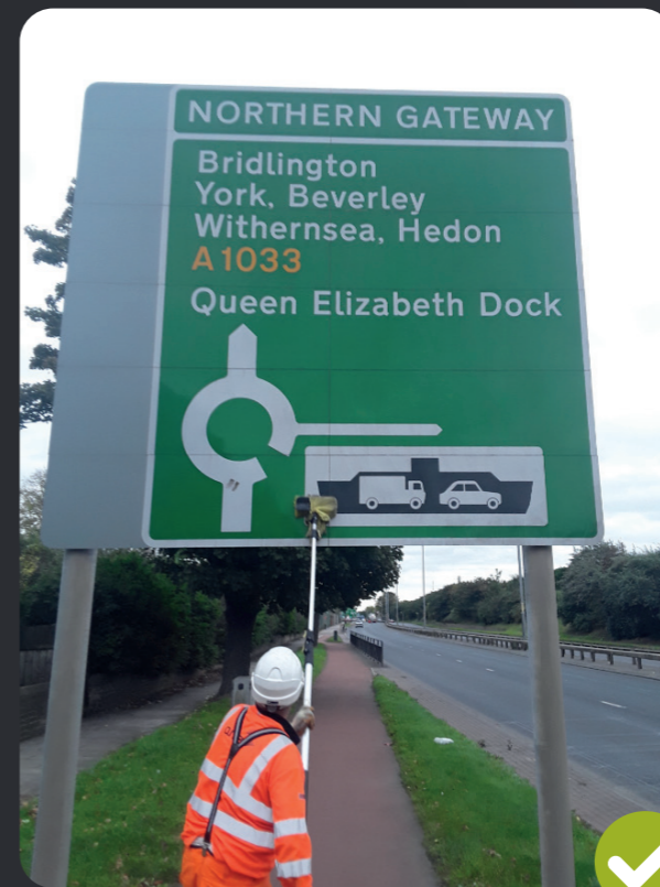
A sign being cleaned in Hull
