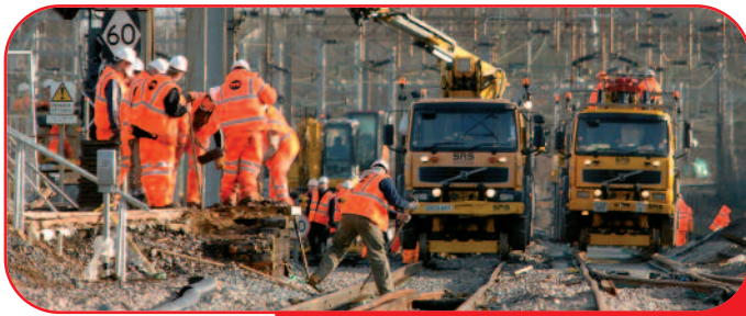
Engineers work to upgrade the line
