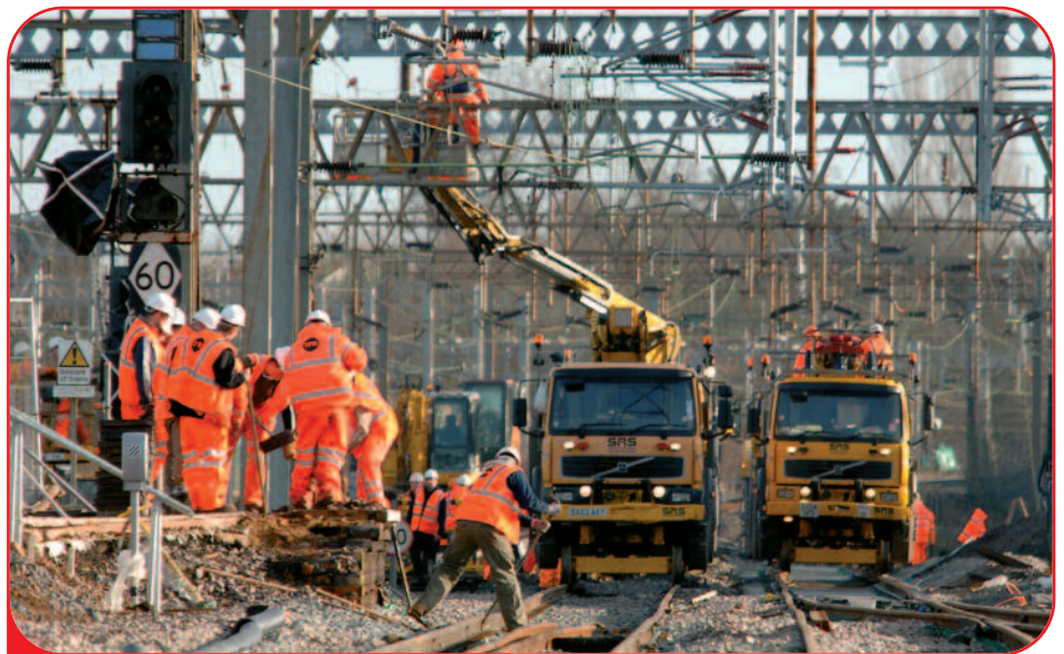
Engineers work to upgrade the line
