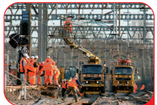
Engineers work to upgrade the line
