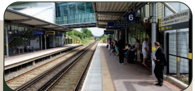
Liverpool South Parkway is a good example of a secure station
