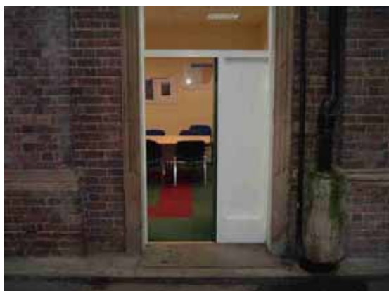
Figure 15 – Meeting room door.
