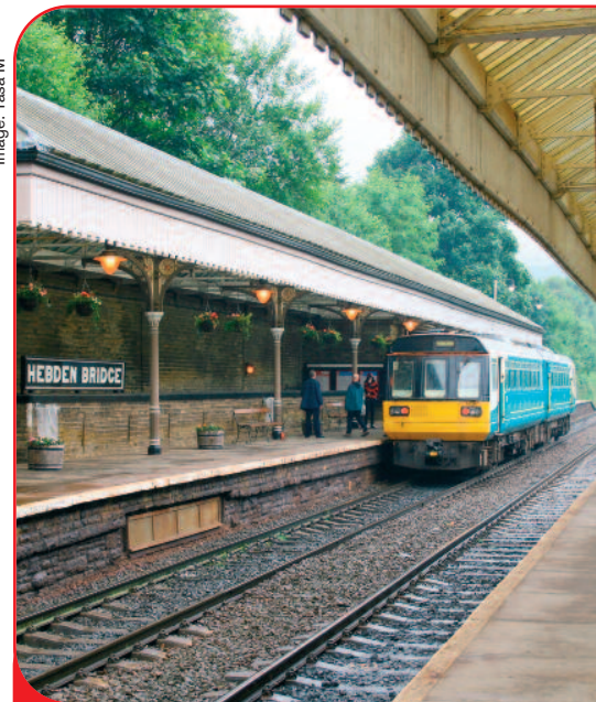
Hebdon Bridge station
