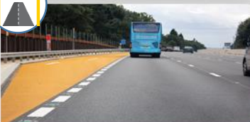
Emergency refuge areas
