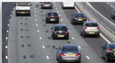
Temporary lane markings
