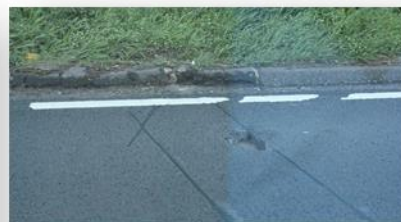
Changes to the road surface
