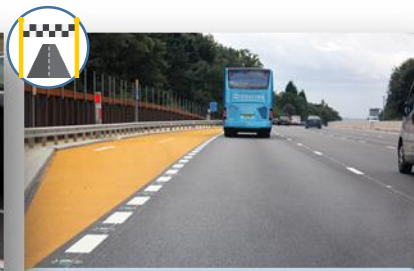
Emergency refuge areas
