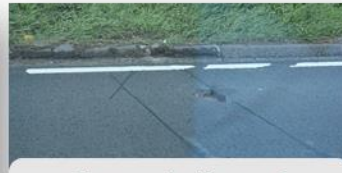
Changes to the road surface
