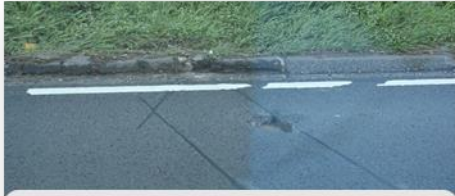
Changes to the road surface
