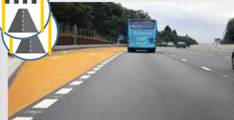
Emergency refuge areas
