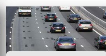
Temporary lane markings
