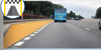
Emergency refuge areas
