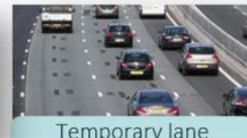
Temporary lane markings
