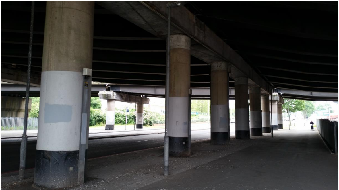
Photo: Pigeon defecation on footpaths under bridges, as seen here under the M5 at Oldbury.
